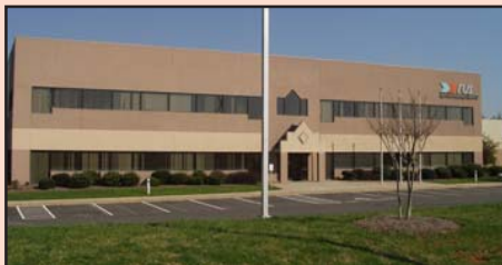
This facade's uninterrupted plane fails to achieve a human-scaled massing. It also has a horizontal orientation rather than a more appropriate series of vertical bays.
