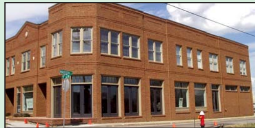
Flat roofs should be screened with a parapet facade on the building's frontage. The parapet should also screen rooftop equipment.
